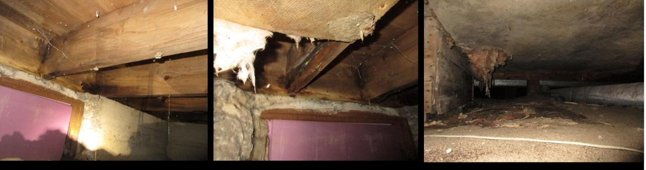
"Moisture rot is present on all visible floor joists at their ends bearing on the foundation. A lost sill plate may have allowed the floor joists to drop 2 inches; and the weight bearing ends, now sitting directly on the cement foundation, are beginning to shear off. This is a major structural concern as shearing floor joists may be pushing outward against the top of the right foundation wall and across the bottom of the right structural wall of the building."
