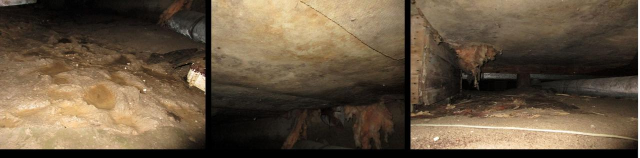
"Extensive building flooding causing evaporation/condensation issues is propagating excessive molds on the underside of the floor structure. The black colored mold is likely Stachybotrys species, the white mold is likely Cladosporium species, and the yellow mold is likely Aspergillus species. ALL areas of floor joists and Homasote (fiber board) attached to the floor joists are saturated wet, and moldy."
