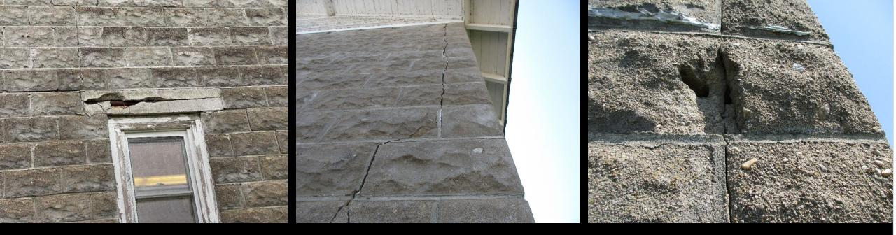
"The step cracking includes mortar joints and through blocks; and continues through the structural concrete apron ledge. This is a structural concern. Step cracking is normally a sign of structural impairment from settling and/or lateral movement. It is your inspector's opinion that this is the result of rotting first floor floor joists shearing from atop the foundation and causing an outward pressure on the top of the foundation and on the base of the exterior structural walls."
